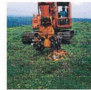
Clearing of stumps
