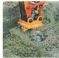
Digging the foundation for electric power pylon
