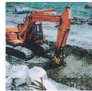
Soft ground improvement work
