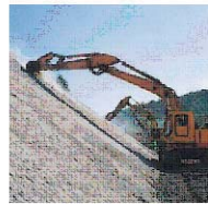
Cutting face of slope
