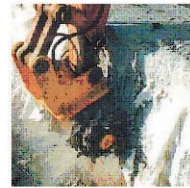
Chipping the concrete surface
